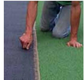
Make sure the 2 halves are placed as close together as possible. There cannot be any overlap! This must be done very precisely, because you want to create a fitted seam. Look at the seam from a number of different angles before joining the strips together.
