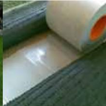
*Unroll the QuickSeam tape and remove the sheet.*
